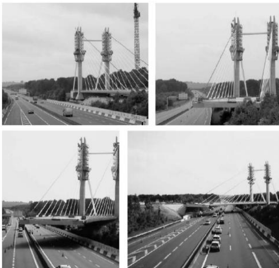
Rasm 12.54 Ko‘prik oraliq qurilmalarini aylantirib qurish misoli (Fraysine)
