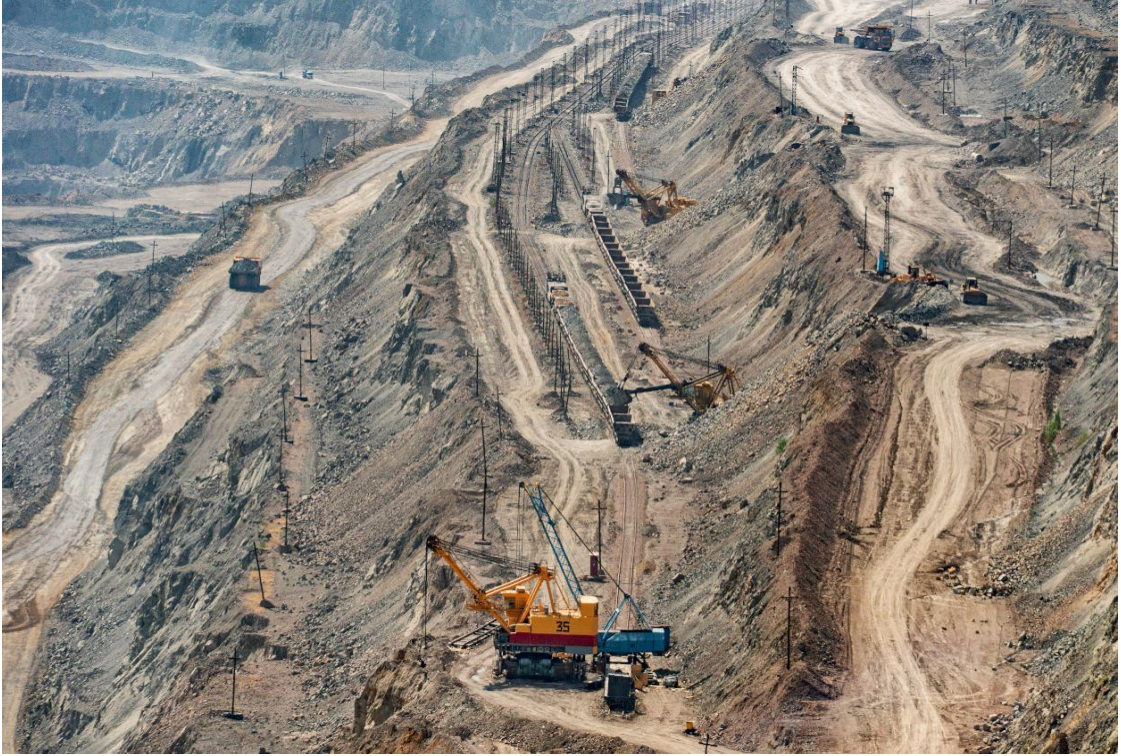
Excavation and loading works (Kalmakyr)
