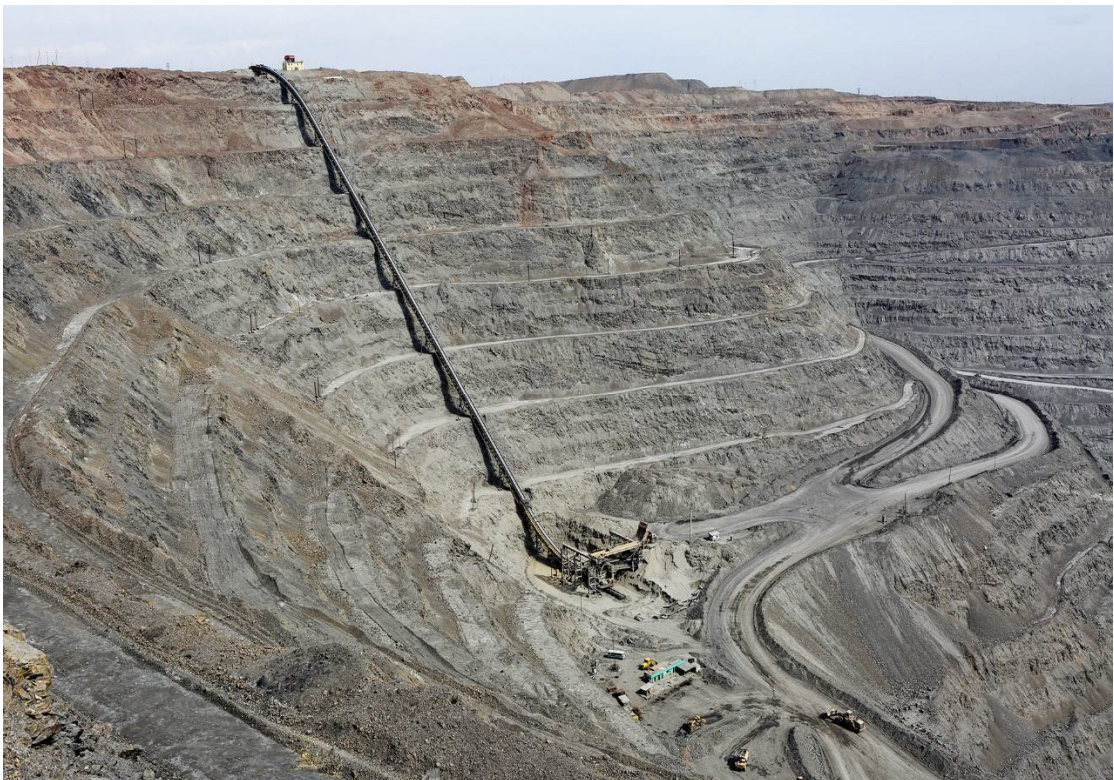
KNK-270 complex (Muruntau steep-slope conveyor)
