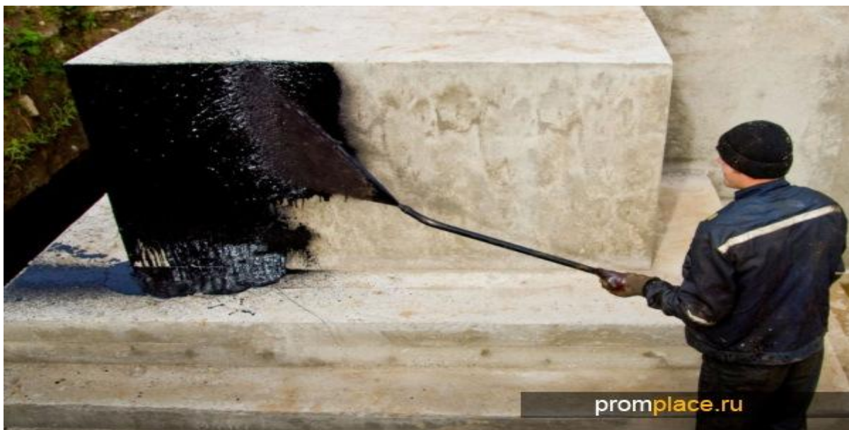
6-rasm. Issiq mastikalarqoplash jarpayon.
