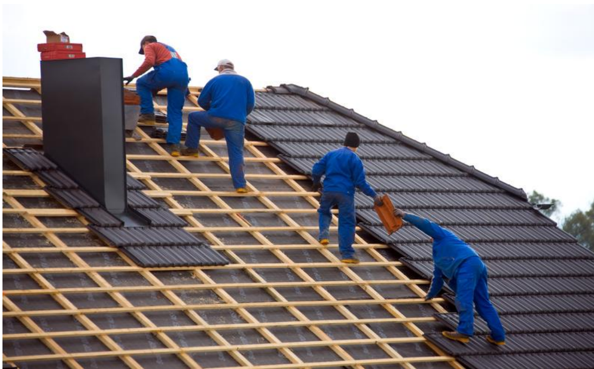
6-rasm. Cherepitsali tomlar terish usullari
