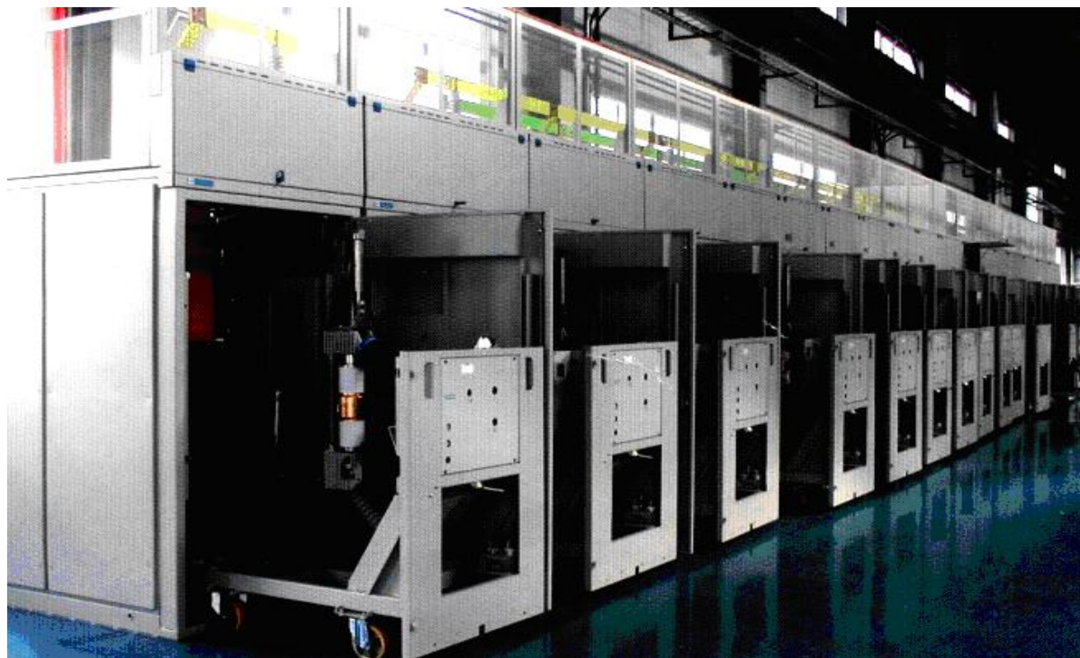
40b-rasm. Fider kameralari KVVO-2.
