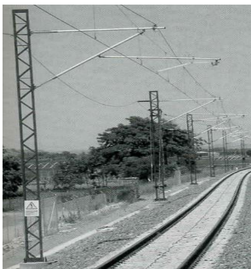
11.5-rasm. Toledo – La-Sagra liniyasida SICAT H1.0 kontakt tarmog‘i
