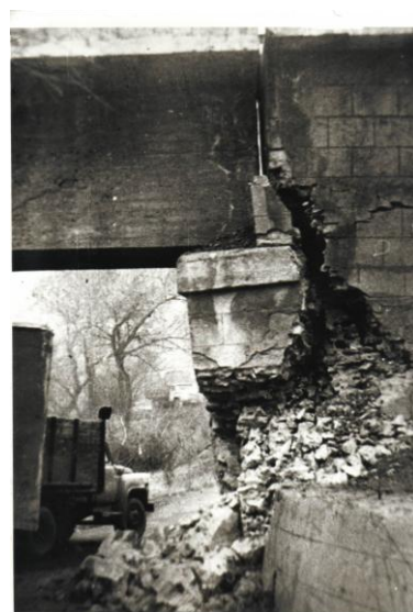
2.1-rasm. 1987 y. Spitak zilzilasi natijasida ko'priklarining tayanchlarining shikastlanishi
