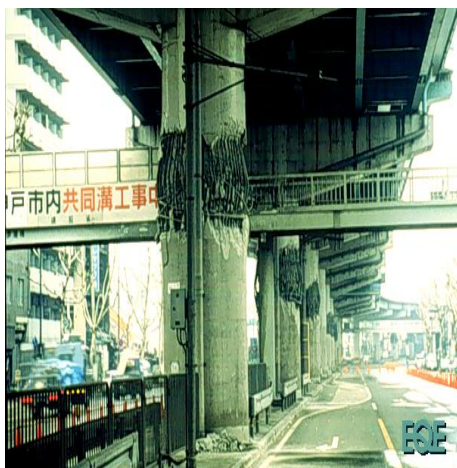
2.3-rasm. 1995 y. Kobo zilzilasi natijasida ko‘prik tayanchlarining shikastlanishi
