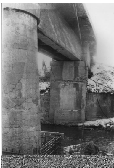
2.1-rasm. 1987 y. Spitak zilzilasi natijasida ko'priklarining tayanchlarining shikastlanishi
