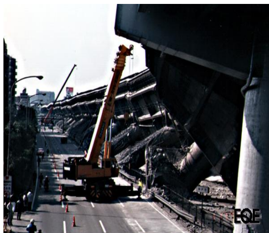
2.3-rasm. 1995 y. Kobo zilzilasi natijasida ko‘prik tayanchlarining shikastlanishi
