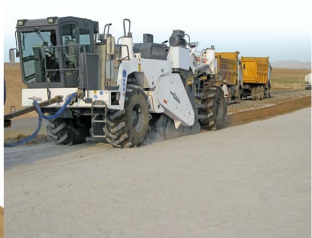
Figure 1.5. Mixing in place using traveling mixing machines (Wirtgen WR 2500).
