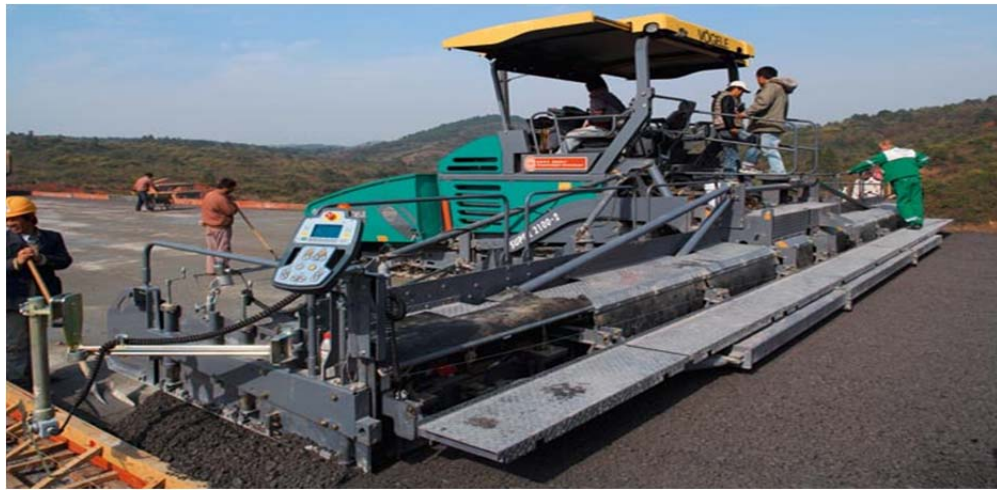
Figure 1.8. Construction using paver machinery (central-mixing-plant)
