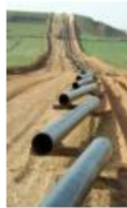
Pipeline under construction
