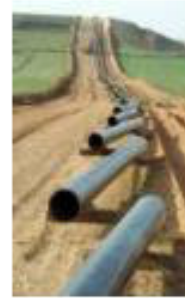
Pipeline under construction
