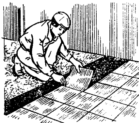
59-rasm. Plitkalarni sovuq mastikada yopishtirish.
