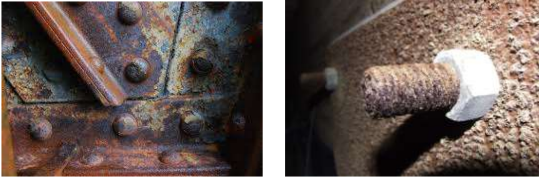
2-Rasm. Metallarda zang ko‘rinishlari
