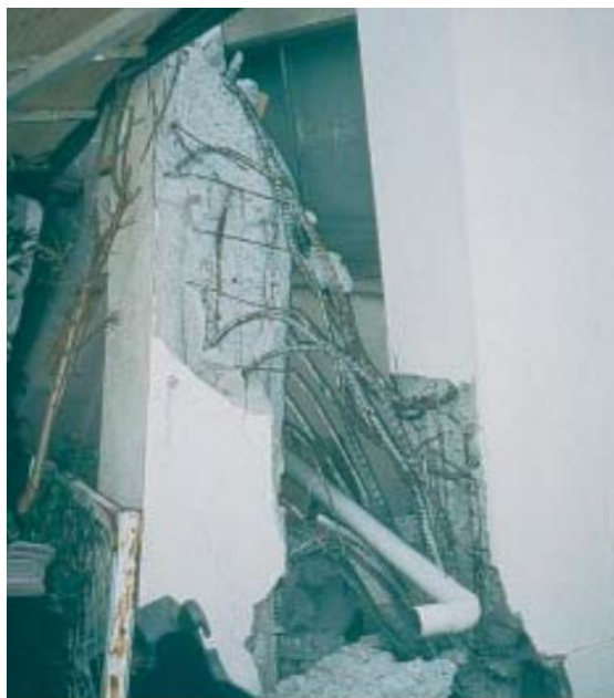
Figure 9.6. ... and these are the remains of the left edge ground floor column (Kobe, Japan 1995).
