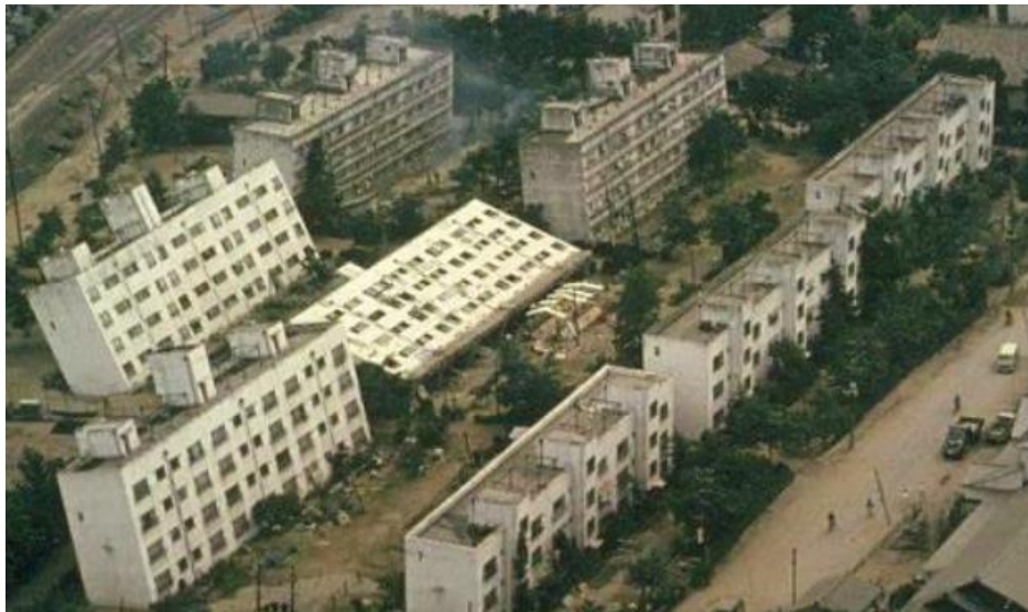
Figure 3.5 Collapsed apartment buildings in the Niigata area of Japan. The material beneath the buildings was liquefied to varying degrees by the 1964 earthquake.
