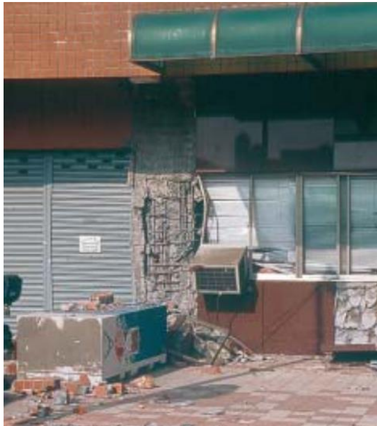
Figure 9.7. ...thanks to resistant columns with well detailed stabilising and confining reinforcement (Taiwan 1999).
