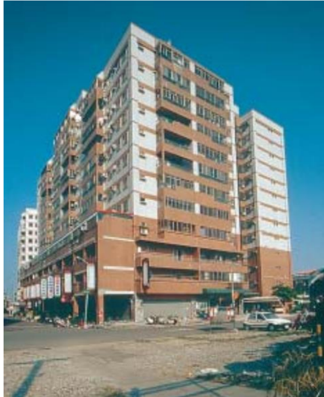
Figure 9.5. This multi-storey building escaped collapse by a hair's-breadth...
