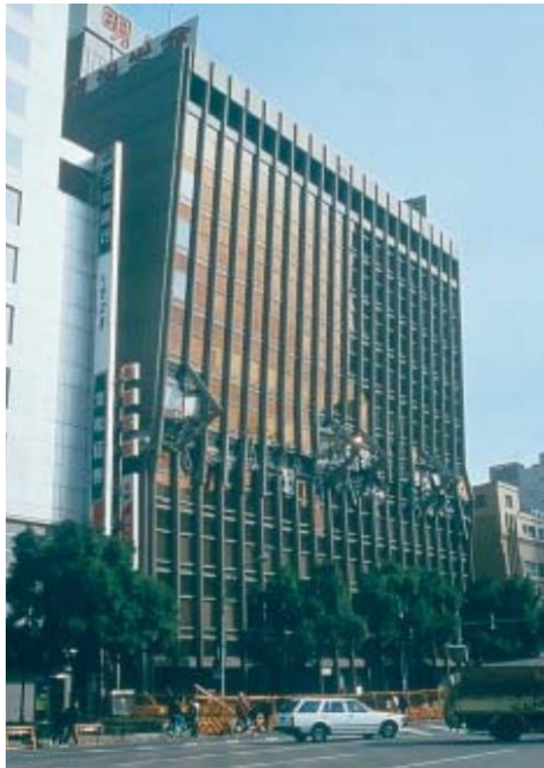
Figure 9.9. In this office building also, an upper storey failed. The top of the building has collapsed onto the floor below, the whole building rotated and leaned forwards.
