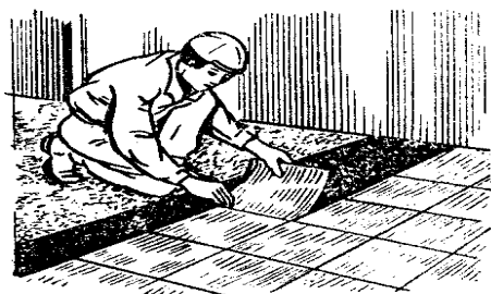
59-rasm. Plitkalarni sovuq mastikada yopishtirish.
