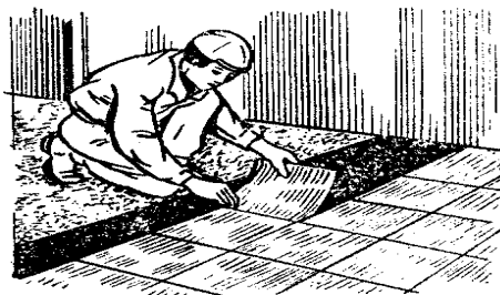
59-rasm. Plitkalarni sovuq mastikada yopishtirish.
