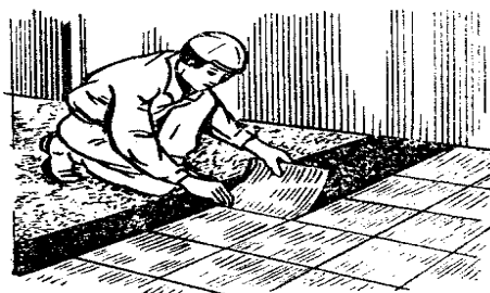
59-rasm. Plitkalarni sovuq mastikada yopishtirish.
