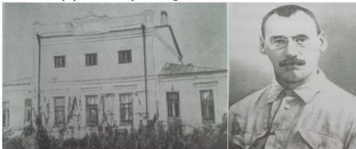
Photo 149, 150. Building of Central breeding station of All Union Scientific-Research Institute (1929) and Gavriil Semenovich Zhaytsev-the first director of Central (former Turkistan) Breeding Station in 1922-1929.
