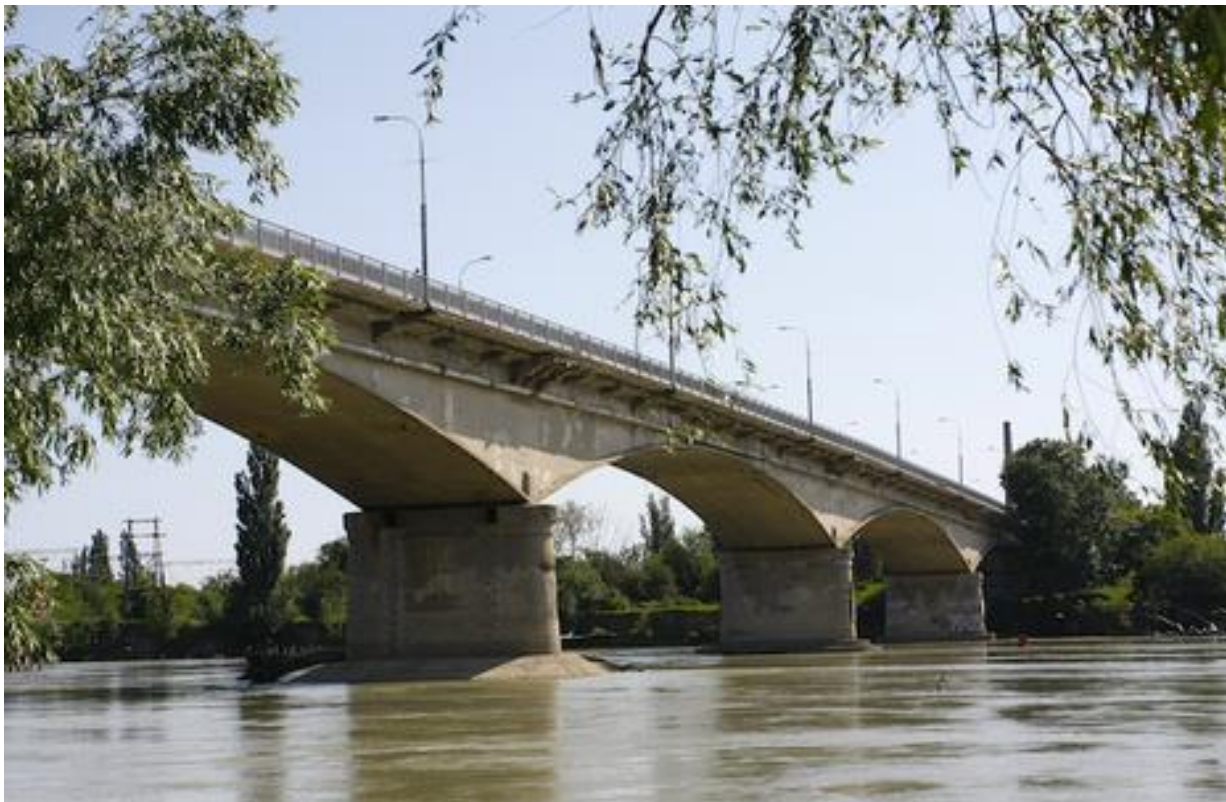
38-rasm. Katta temirbeton ko‘prik
