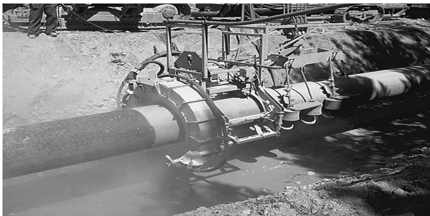
7.5.9-rasm. Yuzani avtomatik tarzda tayyorlash.
