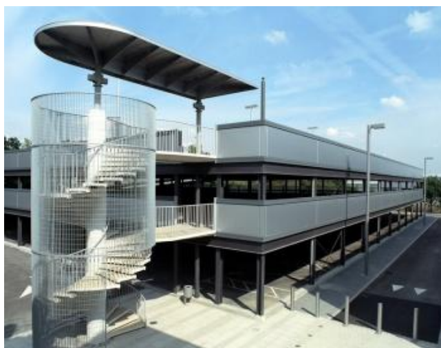
2.3.-расм. Steel-framed, multi-storey car park, Reading (Image courtesy of Bourne Construction Engineering Ltd.)
