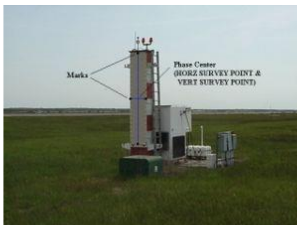
An MLS elevation guidance station.
