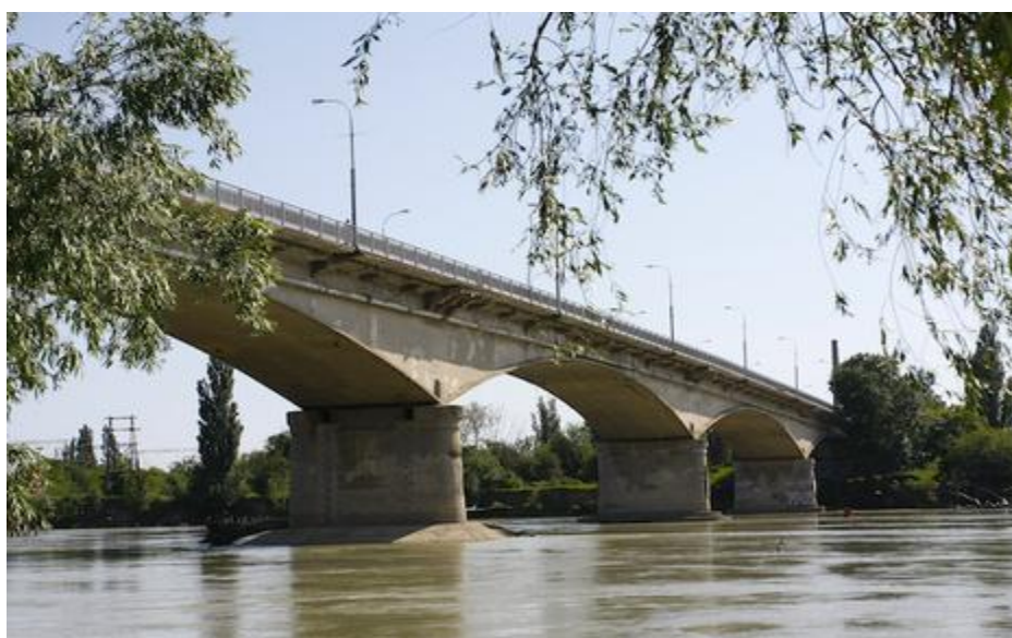
65-rasm. Katta temirbeton ko'prik
