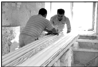
88-rasm. Quyma ganchkorlik ishlarini bajarish.
