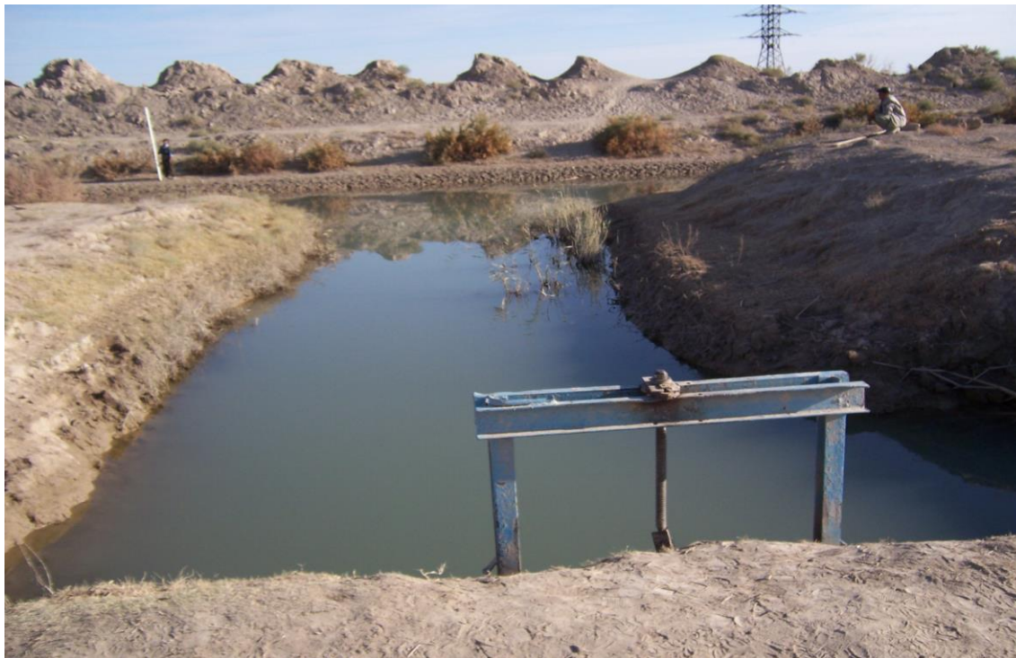
2.3 - rasm. 31 – X - 2 kanaliga suv olish inshooti
