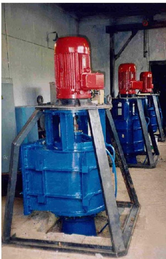
12.5-rasm. 20PrD parrakli diogonal turbinaning o'rnatilish sxemasi (a) hamda ishchi holatidagi ko'rinishi (b)
