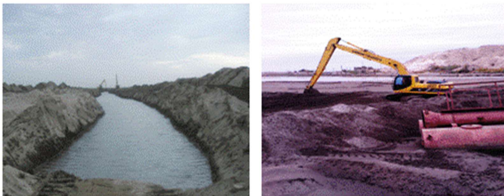
15-rasm. Amudaryodan QMK ga to‘g‘onsiz suv olishda yoriq ochish ishlari.
