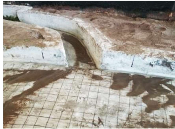
9-rasm. Vaqt o'tishi bilan to'g'onsiz suv olish inshootining kirish qismida nanoslarning to'planishi
