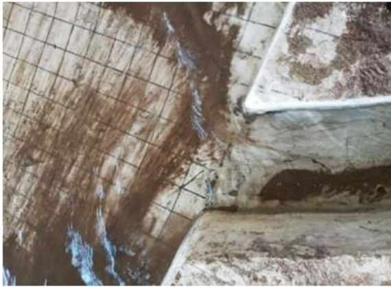
8-rasm. To'g'onsiz suv olish inshootining kirish qismida nanoslarning to'planishi
