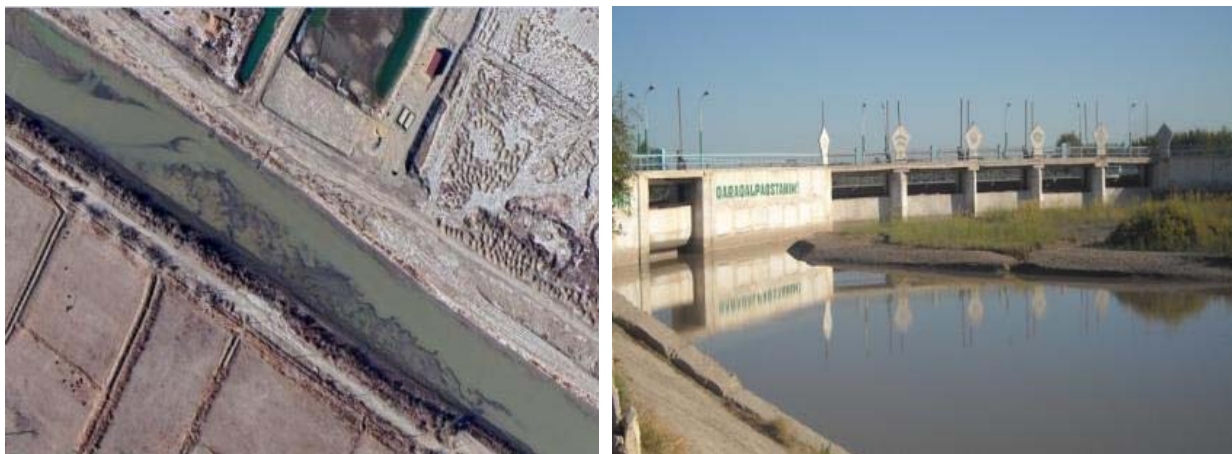
1-rasm. Anasay magistral kanalining loyqa bosishi va yuvilishi
