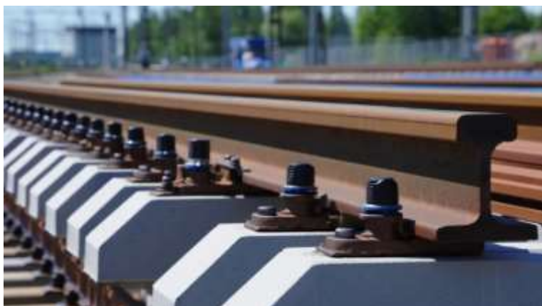
8-rasm. Temir-beton shpallari
