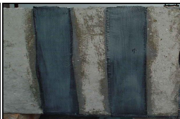
4.17-rasm. To'sin o'ralgan polosaning oxirgi bosqichi
