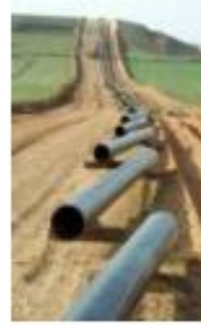
Pipeline under construction
