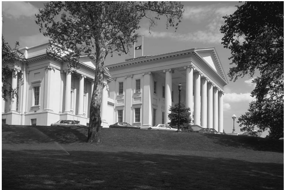
State governments are an important seat of tourism policy formation. Shown here is the state capitol building in Richmond, Virginia. Photo courtesy of Washington, D.C., and the Capital Region.
