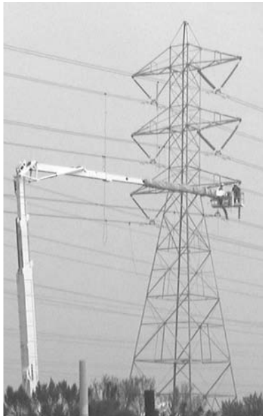
Figure 10-7. Insulated buckets.
