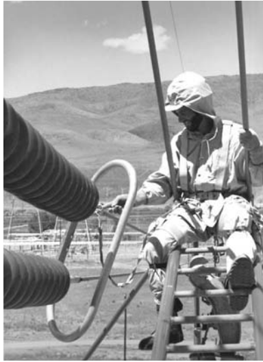
Figure 10-9. Bare-hand, live-line maintenance.
