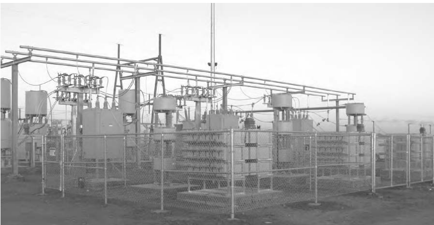
Figure 4-42. Static VAR compensator. Courtesy of Jeff Selman.
