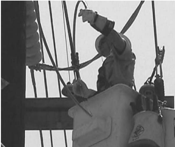
Figure 10-11. Live maintenance distribution. Courtesy of Alliant Energy.
