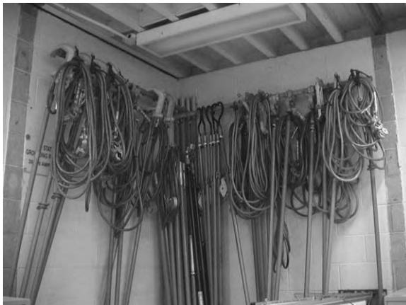
Figure 10-10. Ground jumpers.
