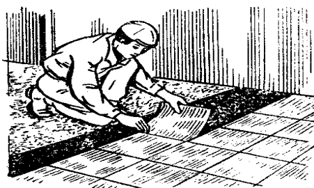
59-rasm. Plitkalarini sovuq mastikada yopishtirish.
