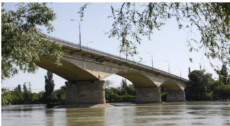
53-rasm. Katta temirbeton ko'prik
