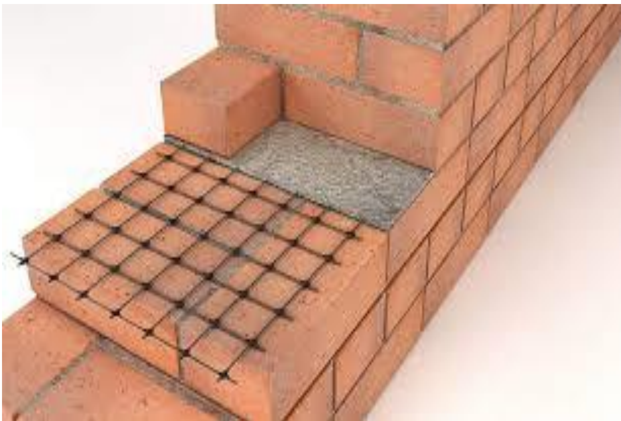
36-rasm. G'ishtni chok bostirish usullari.
