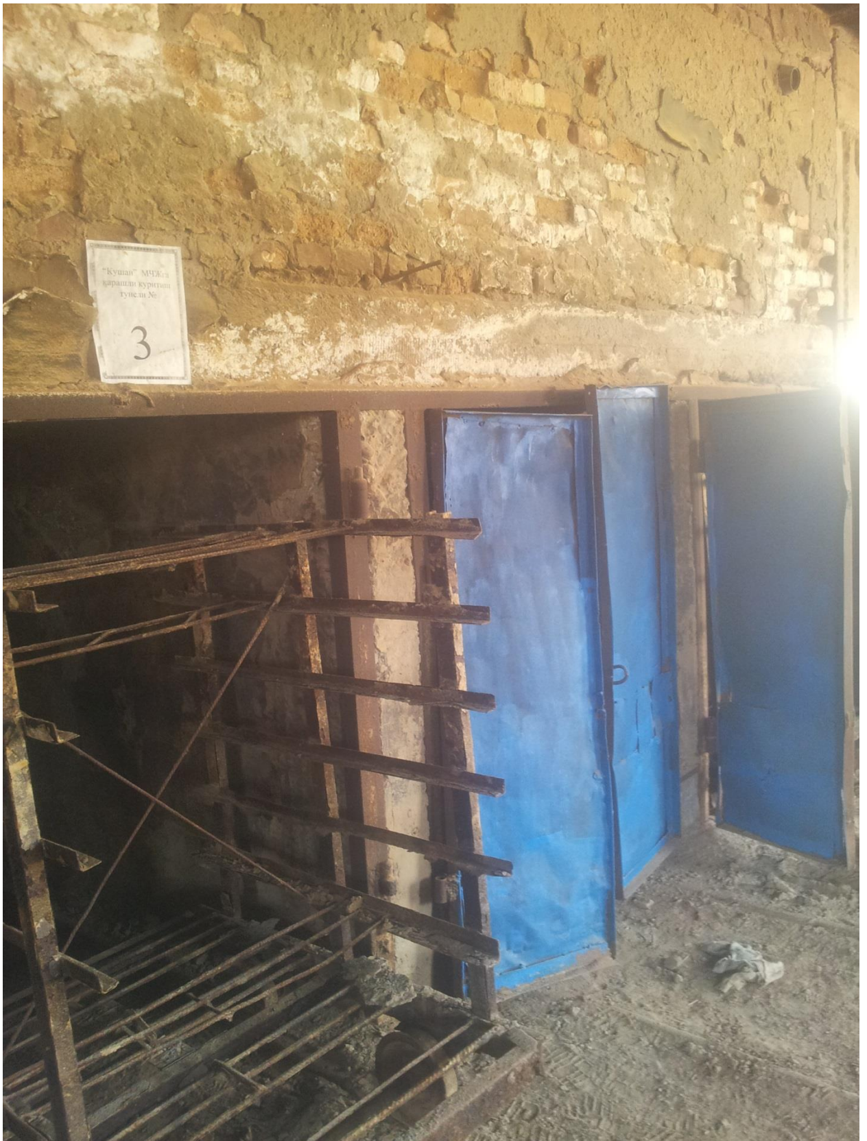
14-rasm. Kushon MFY kushon MCHJga qarashli quritish tunneli.
