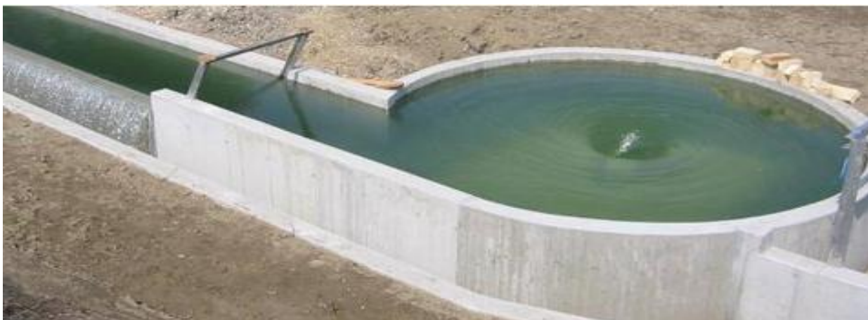
2.15-rasm.GES ning suv girdobining ko'rinishi
