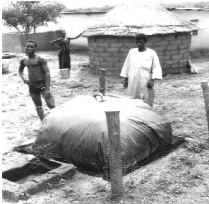
1.2-rasm. 1940-yillarda yaratilgan biogaz qurilmasining ko`rinishi (Misr).
