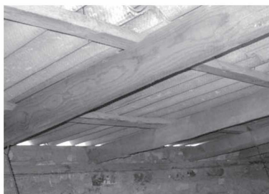
1.58-rasm. Chordoqli tomda to'sinning tagsinchiga, panjara (obreshyotka)ning to'singa o'rnatilishi.
