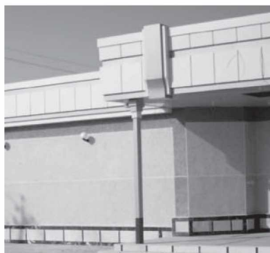
1.30-rasm. Devorning poypeshi marmardan, karnizi zamonaviy materialdan (alumin profildan) ishlanishi.
