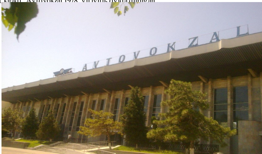
1-rasm. Toshkent avtovokzali Chipta sotish kassasi:
